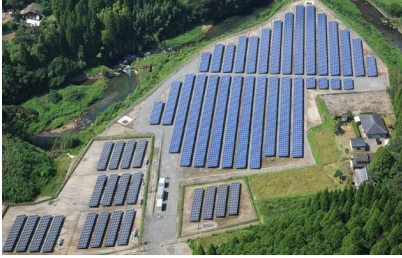
S-01 CS Shibushi-shi Power Plant 1.2MW
