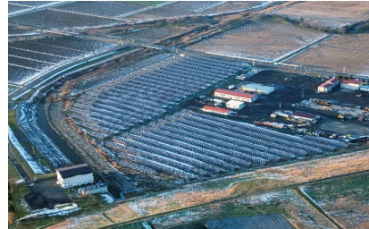
S-22 CS Ishikari Shinshinotsu-mura Power Plant 2.3MW
