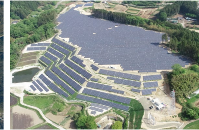
S-25 CS Ogawara-machi Power Plant 7.5MW
