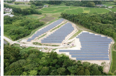
S-23 CS Osaki-shi Kejonuma Power Plant 0.9MW
