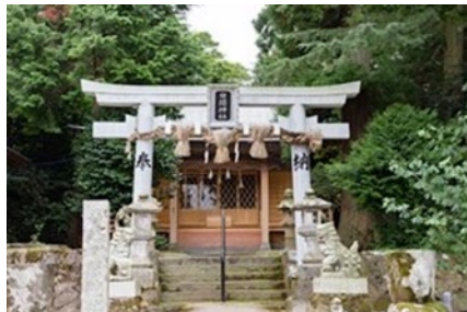
Repaired the Hima Jinja Shrine
