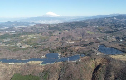
S-21 CS Izu-shi Power Plant 10.7MW
