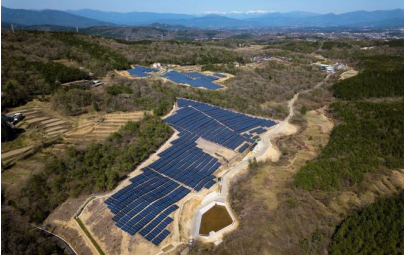
S-16 CS Ena-shi Power Plant 2.1MW
