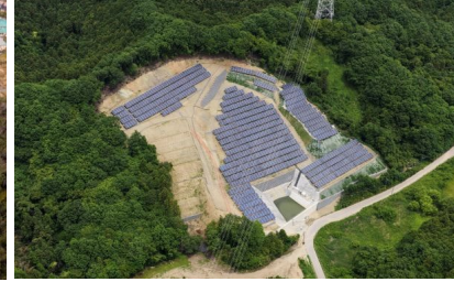
S-19 CS Misato-machi Power Plant 1.1MW
