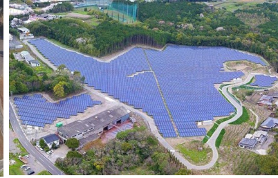
S-10 CS Minami Shimabara-shi Power Plant (East & West) 3.9MW
