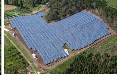
S-04 CS Isa-shi Dai-ni Power Plant 2.0MW
