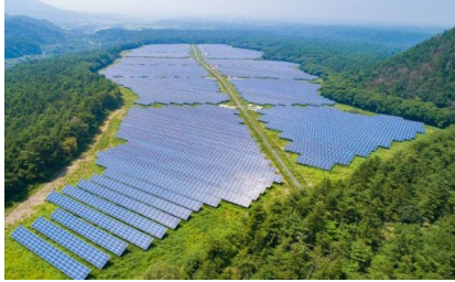
S-17 CS Daisen-cho Power Plant (A&B) 27.3MW
