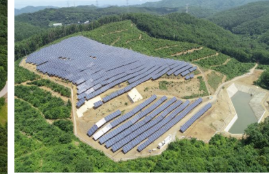
S-20 CS Marumori-machi Power Plant 2.2MW
