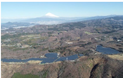
S-21 CS Izu-shi Power Plant 10.7MW
