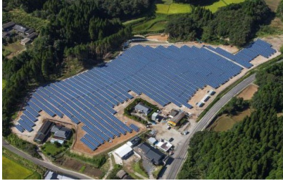
S-06 CS Isa-shi Dai-san Power Plant 2.2MW
