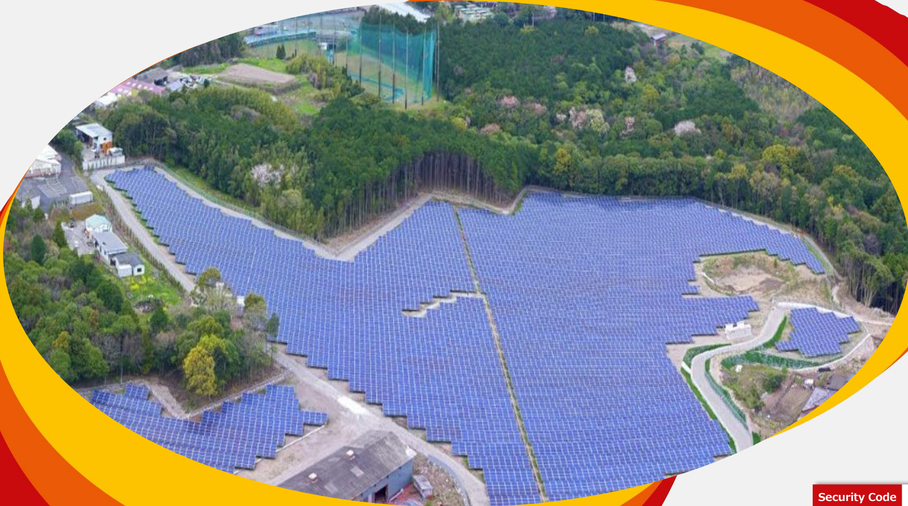
S-10 CS Minami Shimabara-shi Power Plant (east) (west)
