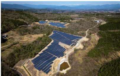
S-16 CS Ena-shi Power Plant 2.1MW
