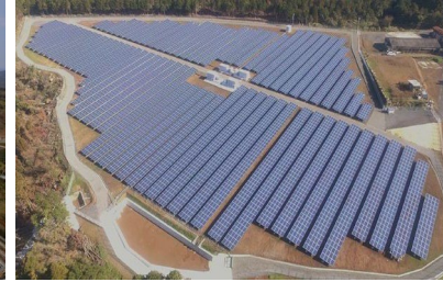
S-09 CS Ashikita-machi Power Plant 2.3MW
