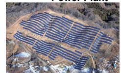
S-11 CS Minano-machi Power Plant
