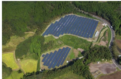
S-05 CS Yusui-cho Power Plant
