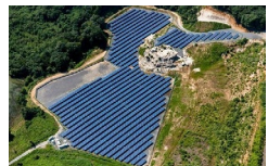
S-07 CS Kasama-shi Dai-ni Power Plant
