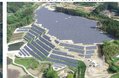
S-25 CS Ogawara-machi Power Plant 7.5MW
