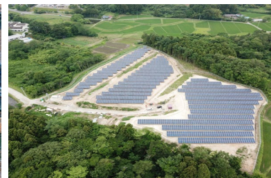
S-23 CS Osaki-shi Kejonuma Power Plant 0.9MW
