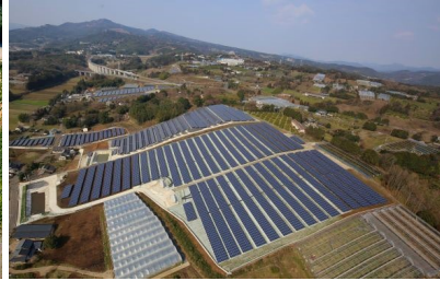
S-08 CS Hiji-machi Power Plant 2.6MW
