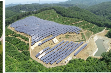
S-20 CS Marumori-machi Power Plant 2.2MW
