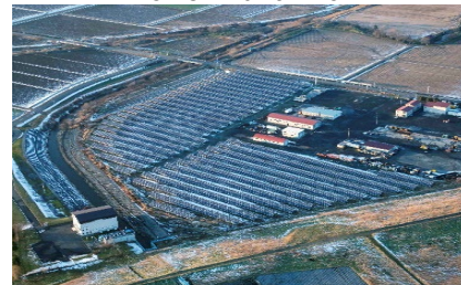
S-22 CS Ishikari Shinshinotsu-mura Power Plant 2.3MW
