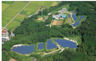
S-12 CS Kannami-cho Power Plant 1.3MW
