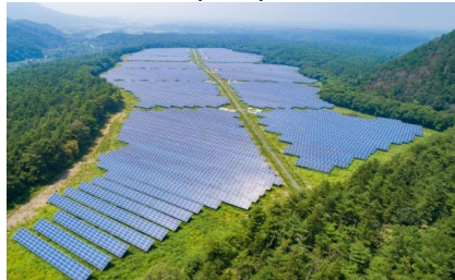
S-17 CS Daisen-cho Power Plant (A&B) 27.3MW
