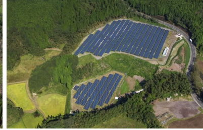
S-05 CS Yusui-cho Power Plant 1.7MW
