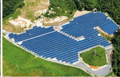
S-03 CS Kasama-shi Power Plant 2.1MW
