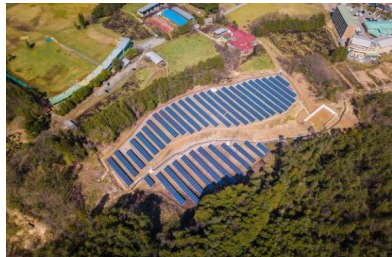
S-18 CS Takayama-shi Power Plant 1.0MW
