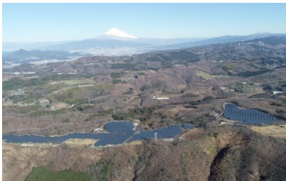
S-21 CS Izu-shi Power Plant 10.7MW
