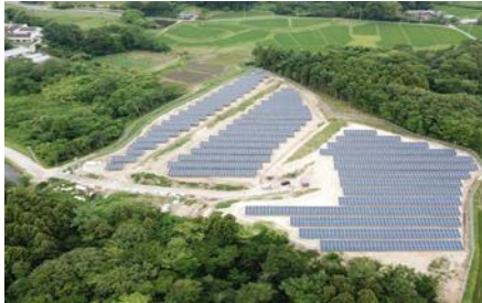
S-23 CS Osaki-shi Kejonuma Power Plant 0.9MW
