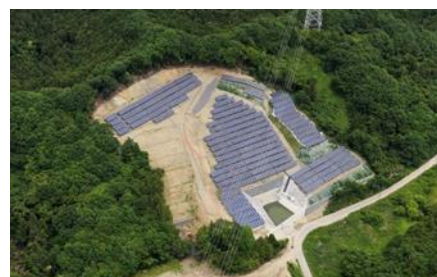
S-19 CS Misato-machi Power Plant 1.1MW
