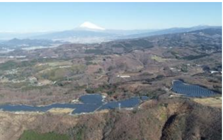
S-21 CS Izu-shi Power Plant 10.7MW
