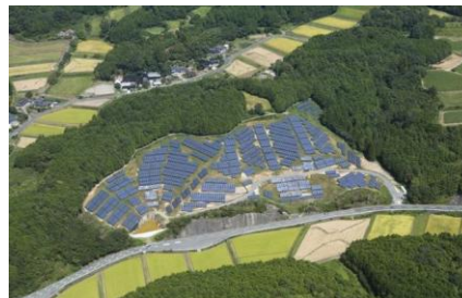
S-15 CS Tsuyama-shi Power Plant 2.0MW
