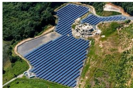
S-07 CS Kasama-shi Dai-ni Power Plant 2.1MW
