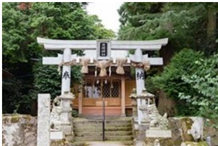
Repaired the Hima Jinja Shrine
