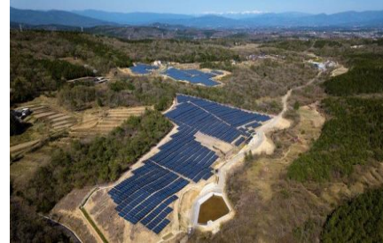
S-16 CS Ena-shi Power Plant 2.1MW
