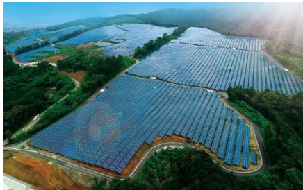
S-13 CS Mashiki-machi Power Plant 47.7MW
