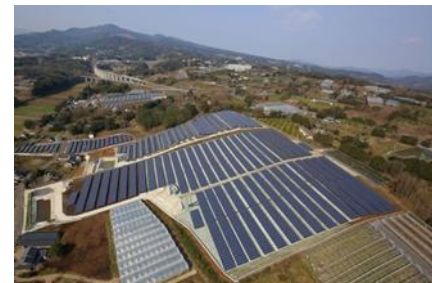
S-08 CS Hiji-machi Power Plant 2.6MW
