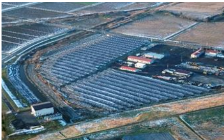
S-22 CS Ishikari Shinshinotsu-mura Power Plant 2.3MW
