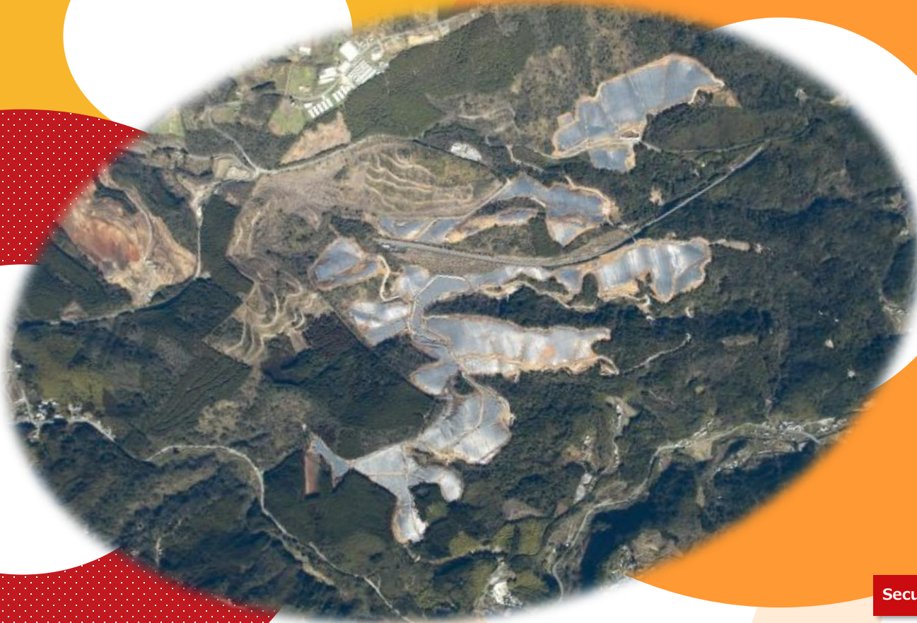
S-24 CS Hiji-machi Dai-ni Power Plant
