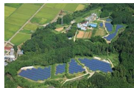
S-12 CS Kannami-cho Power Plant 1.3MW
