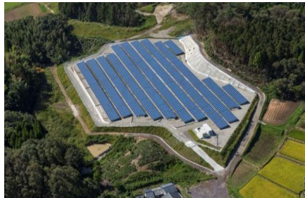
S-02 CS Isa-shi Power Plant 0.9MW
