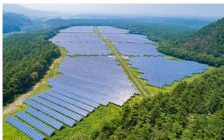
S-17 CS Daisen-cho Power Plant (A&B) 27.3MW
