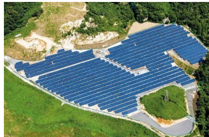
S-03 CS Kasama-shi Power Plant 2.1MW
