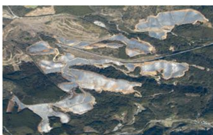
S-24 CS Hiji-machi Dai-ni Power Plant 53.4MW
