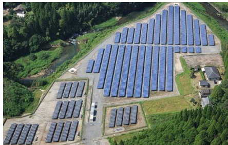
S-01 CS Shibushi-shi Power Plant 1.2MW
