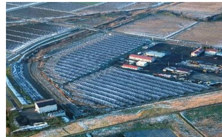
S-22 CS Ishikari Shinshinotsu-mura Power Plant 2.3MW
