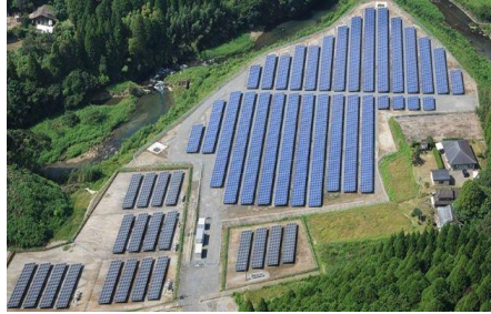
S-01 CS Shibushi-shi Power Plant 1.2MW
