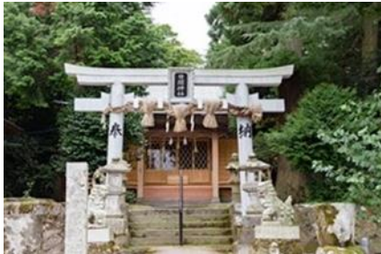
Repaired the Hima Jinja Shrine
