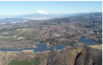
S-21 CS Izu-shi Power Plant 10.7MW
