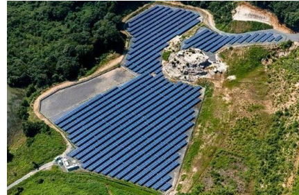
S-07 CS Kasama-shi Dai-ni Power Plant 2.1MW
