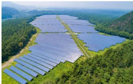
S-17 CS Daisen-cho Power Plant (A&B) 27.3MW
