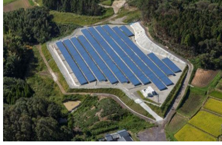
S-02 CS Isa-shi Power Plant 0.9MW
