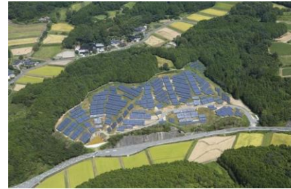
S-15 CS Tsuyama-shi Power Plant 2.0MW
