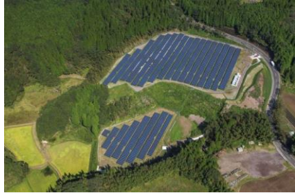
S-05 CS Yusui-cho Power Plant 1.7MW
