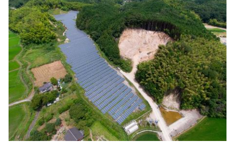
S-28 CS Kama-shi Power Plant 2.2MW
