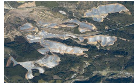
S-24 CS Hiji-machi Dai-ni Power Plant 53.4MW
