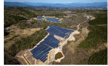
S-16 CS Ena-shi Power Plant 2.1MW
