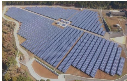
S-09 CS Ashikita-machi Power Plant 2.3MW
