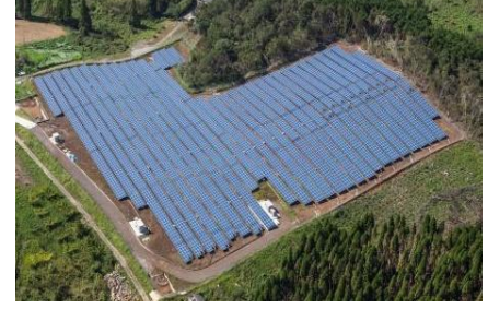
S-04 CS Isa-shi Dai-ni Power Plant 2.0MW
