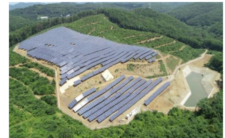
S-20 CS Marumori-machi Power Plant 2.2MW
